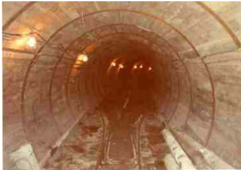
8-foot tunnel with ringbeams and wood lagging
