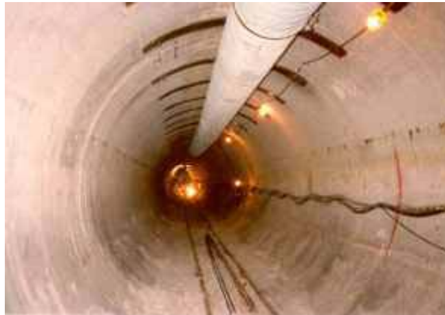
12.5-diameter tunnel with mine mats and rockbolts
